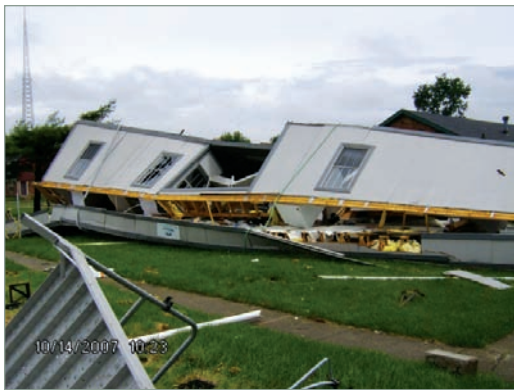
Tornado damage in Indiana
